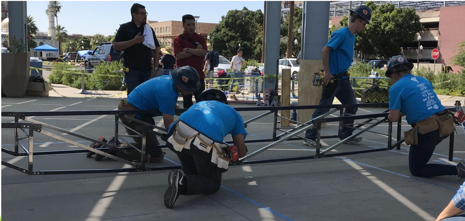
Figure 13: Bridge Construction over river [2]
